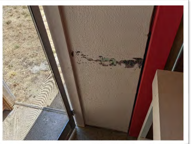
Sample 22-082A.138, Texture/Mastic, Non-ACM
