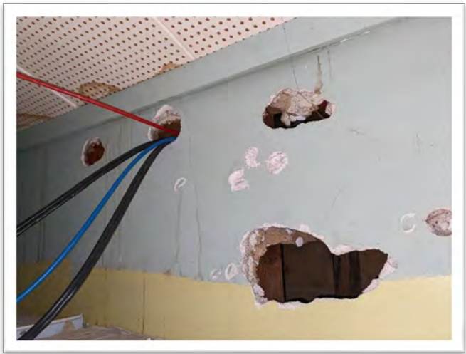
Sample 22-082A.101, Wallboard, <1% Asbestos
