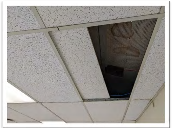
Sample 22-082A.99, 2x4 Ceiling Tile, Non-ACM Sample 22-082A.100, 12" Ceiling Tile, Non-ACM
