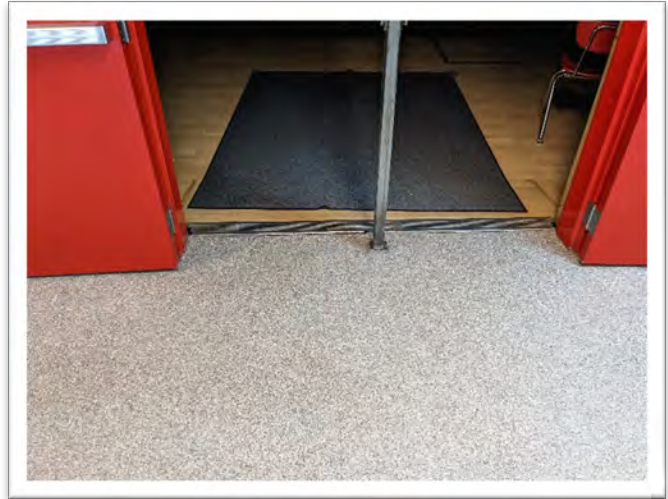
Sample 22-082A.30, Floor Covering, Non-ACM
