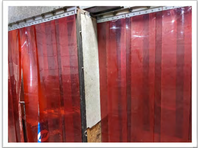
Sample 22-082A.119, Cement Board, 30% Asbestos
