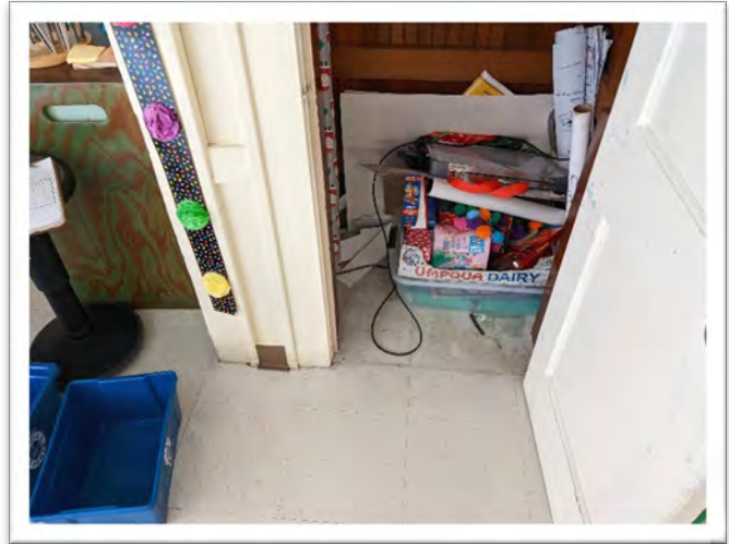
Sample 22-082A.2, Vinyl Floor, Non-ACM Sample 22-082A.3, Cove Base, Non-ACM
